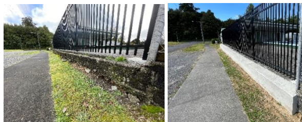
Before and after photos of the pool wall
