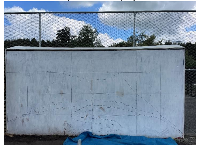
The ball wall is readied for the first coat
