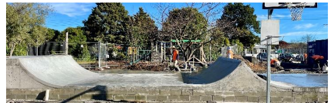
The final concrete pour to finish off the base is happening
