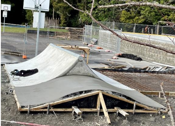
The last of the features are being concreted
